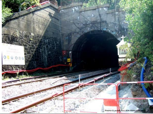
a Improve the loading gauge to P400
